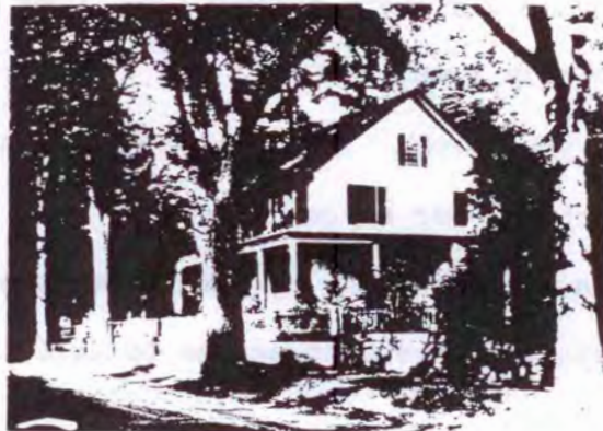
THE HOUSE IN "HIGH ROCK" (18 COMPO RD. WESTPORT, CONN)
